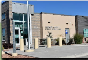
The Fremont County Riverton Justice Center, located in Riverton, Wyoming houses the circuit court for the 9th Judicial District, Fremont County (Riverton)
