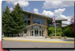
The Teton County Courthouse, located in Jackson, Wyoming houses both the district and circuit courts for the 9th Judicial District, Teton County
